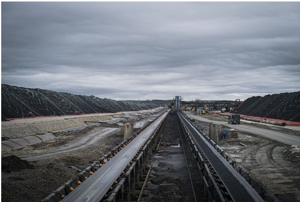
A mining operation in Finland, whose roller conveyor for mined ore is shown, provides nickel for electric-car batteries. PHOTO: ALESSANDRO RAMPAZZO/AGENCE FRANCE-PRESSE/GETTY IMAGES
